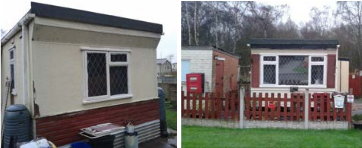
Figure 5.2 Park Home prior to installation of external wall insulation
