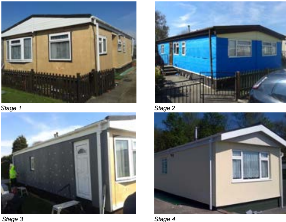
Figure 1.10 Installing EWI on park homes
