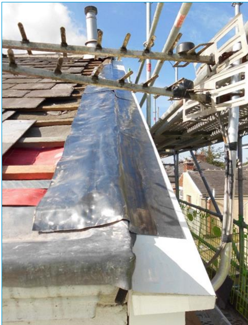
Figure 12 – Ongoing works at top level typical detail of the lead overlap the trim
