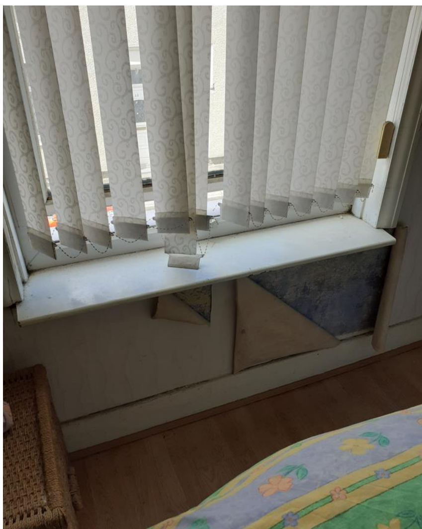
Figure 4 - Cold bridging under the windows due to uneven distribution of the Cavity Wall Insulation
