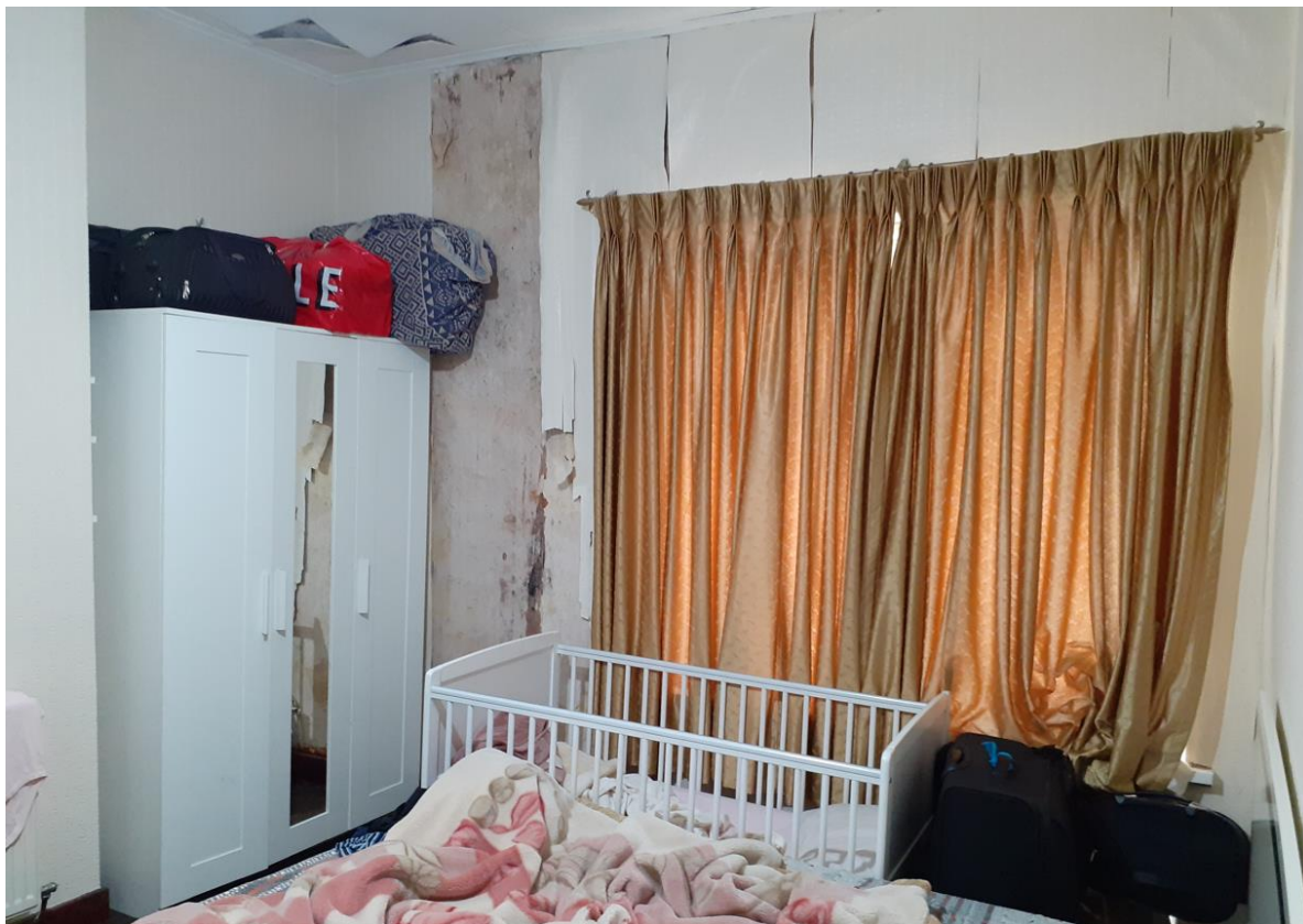
Figure 5 - Wallpaper and ceiling panels falling due to the high condensation and moisture in the fabric
