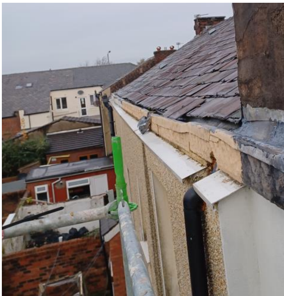
Figure 1 - Typical top-level detail of the 2013 insulation
