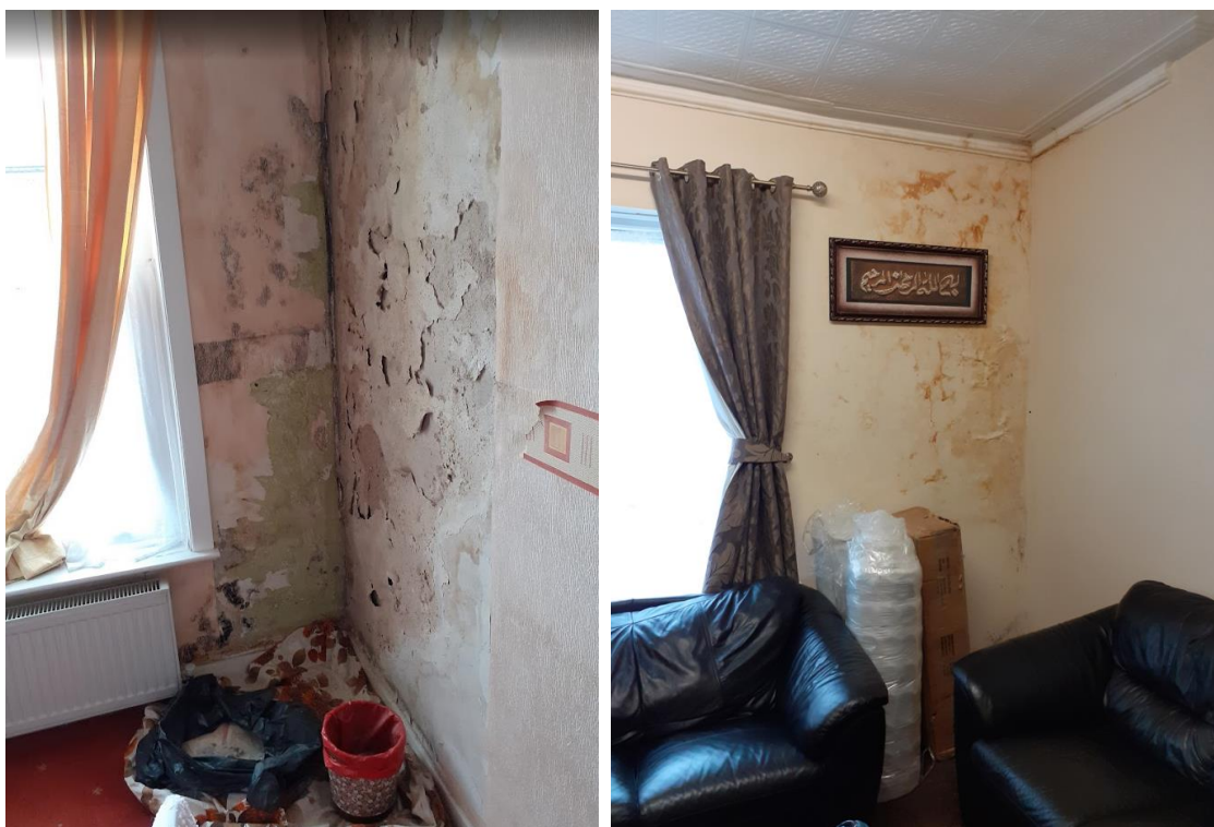
Figure 6 - The plaster would crumble in the most serious water ingress cases.
