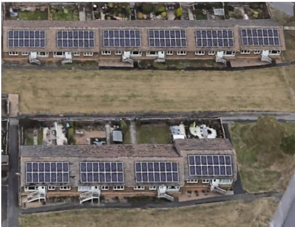
Figure 2.3 Example of terraced bungalows with installations (image from Google Earth)
