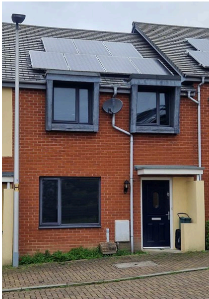
Figure 4.27 Property with 1.75kW solar PV system
