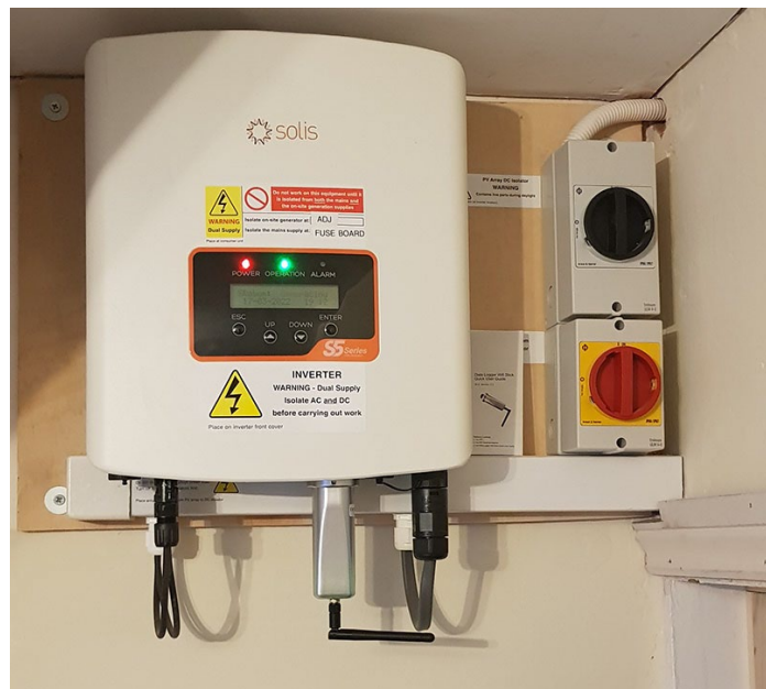
Figure 2.5 (a) Solis Wi-Fi dongle (b) Solis Wi-Fi dongle fitted to Solis inverter
