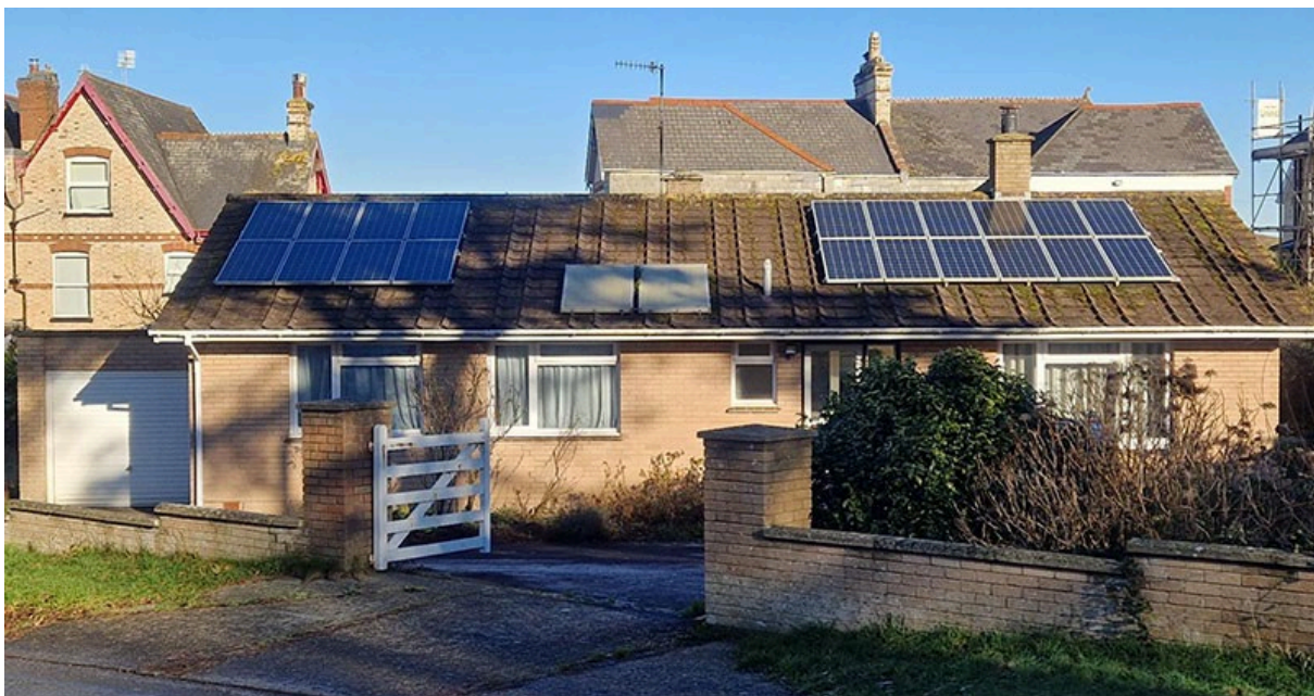
Figure 4.2 Household W-01 with solar PV arrays on the left and right and 2 flat-pate solar thermal collectors in the middle of the roof
