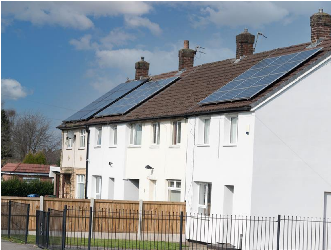
Figure 7.4 Example of Solar PV installation in Stockport
