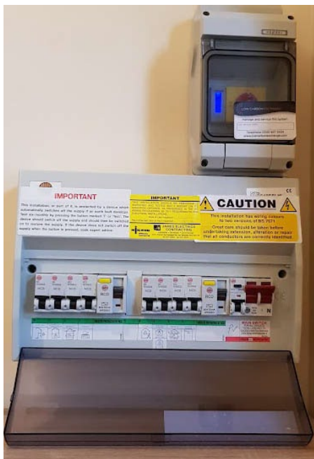
Figure 7.3 AC isolator and generation meter in an enclosure above the consumer unit
