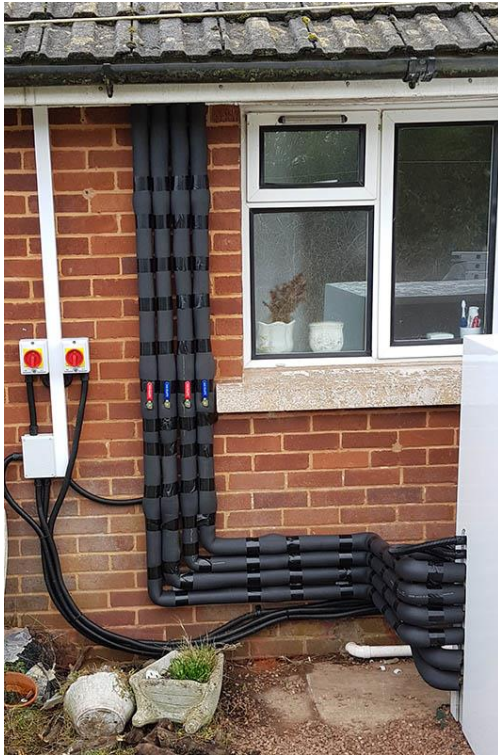
Figure 4.59 AC isolators and pipework for Boxergy Hero system
