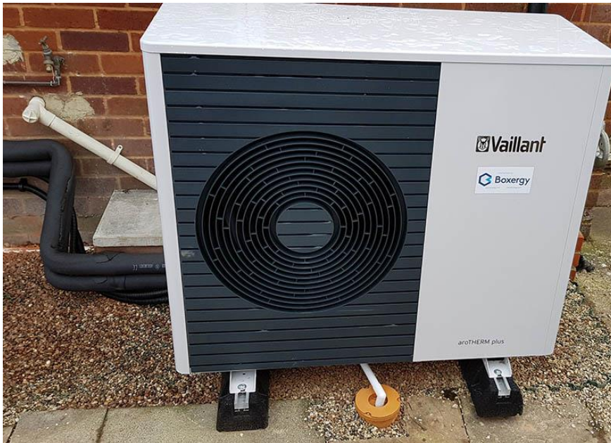
Figure 3.4 Vaillant aroTHERM plus 7kW air-source heat pump
