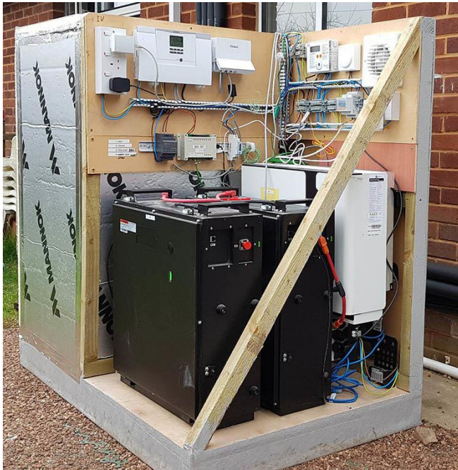
Figure 3.7 Boxergy Hero unit with an Alpha ESS Smile 5 hybrid inverter and 2 x SMILE-BAT-5.7
