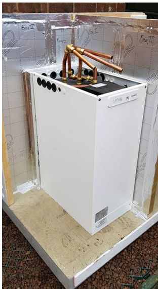
Figure 3.8 Sunamp 3 rd generation UniQ heat battery (in Hero Box and schematic diagram) 13
