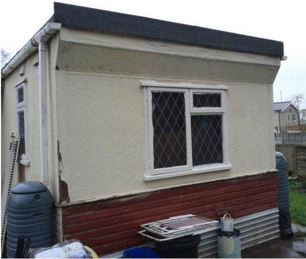
Figure 5.2 Park Home prior to installation of external wall insulation
