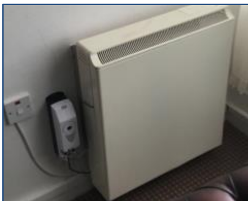
Figure 3.1 a VCharge unit installed in a resident's property
