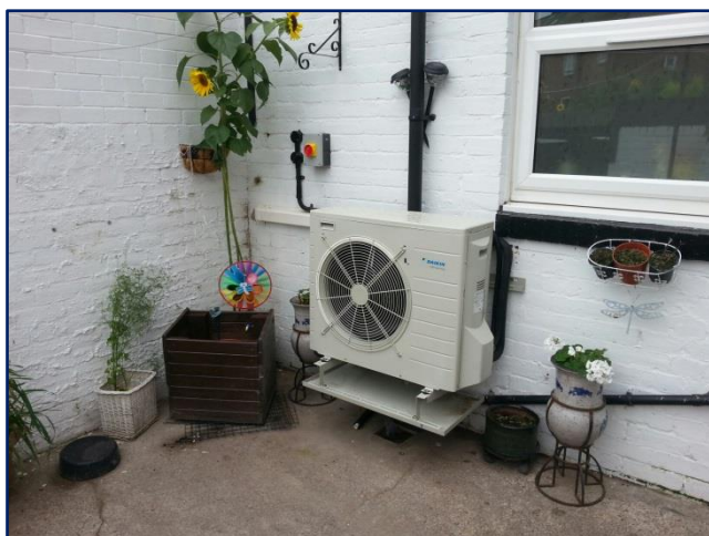
Figure 3.2 External condensing unit
