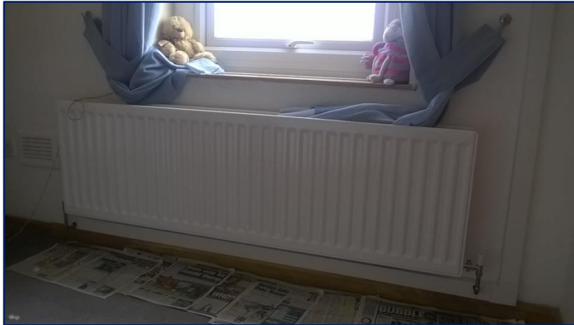
Figure 3.3 Oversized radiators
