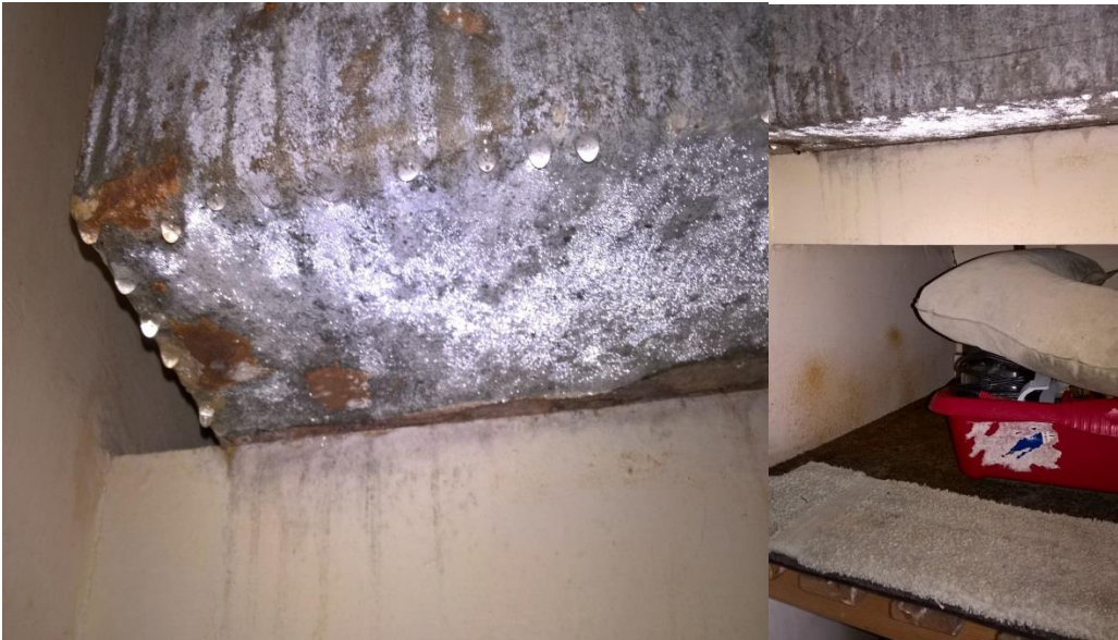
Figure 2.13 Cold water tank causing damp / water ingress.
