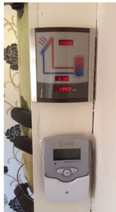
Figure 3.3 (a) left, heat meter installed on a multi-fuel stove system and (b) right, a solar thermal display unit.
