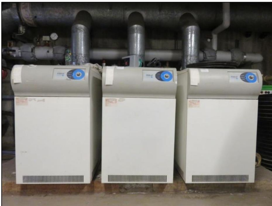
Figure 1-1, 3 gas boilers previously used for the communal heating system
