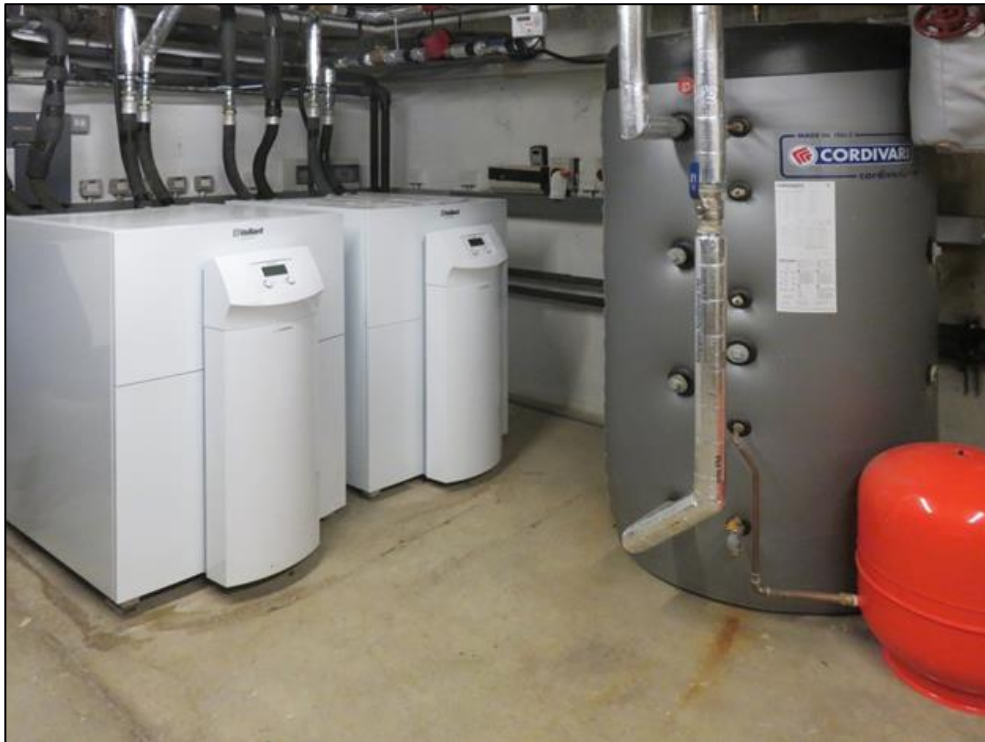
Figure 1-2, Two Vaillant geoTHERM pre-heating GSHPs and buffer tank
