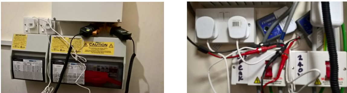
Figure 4.6 showing examples of loggers on the same circuit
