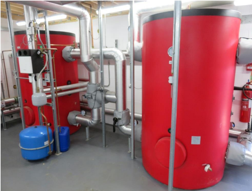
Figure 3.4: two 1500 litre buffer tanks in the plant room
