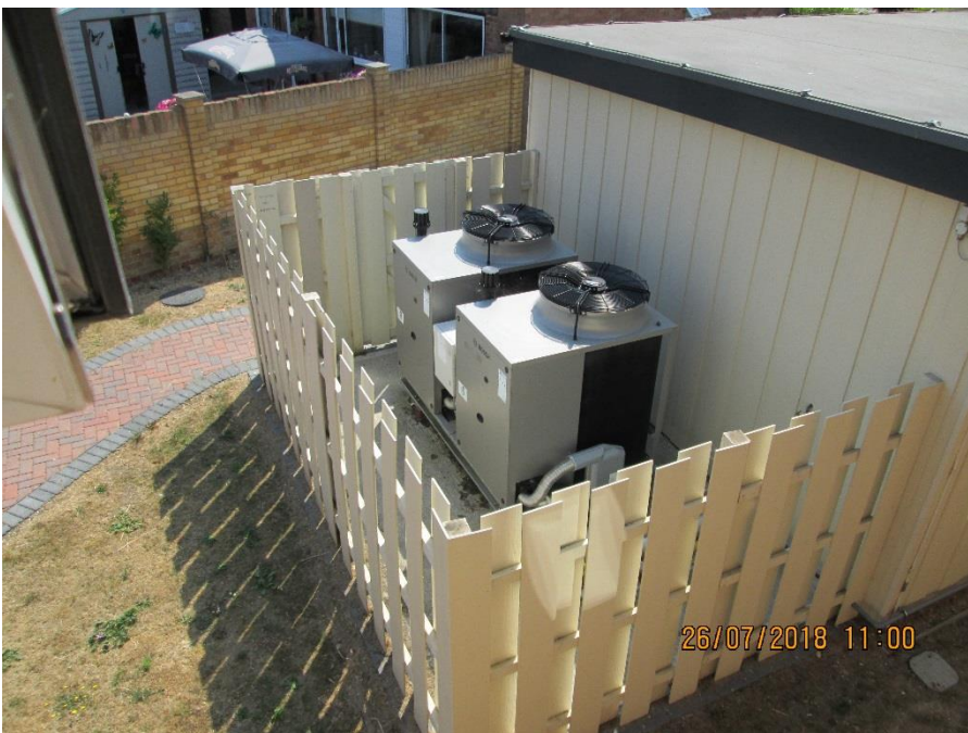
Figure 3.3 Worcester Bosch GAHPs in their compound
