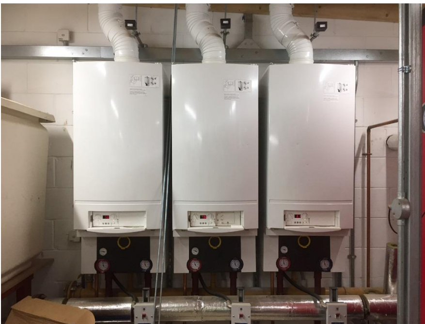
Figure 3.5: three Worcester Bosch back up boilers
