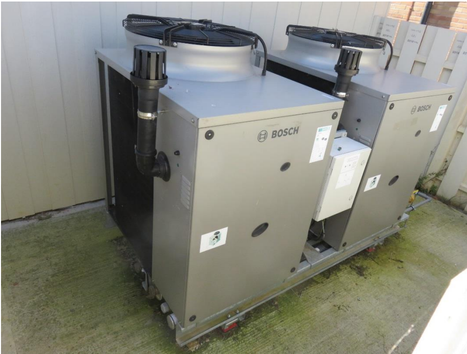
Figure 3.2 view of the two Worcester Bosch GAHPs
