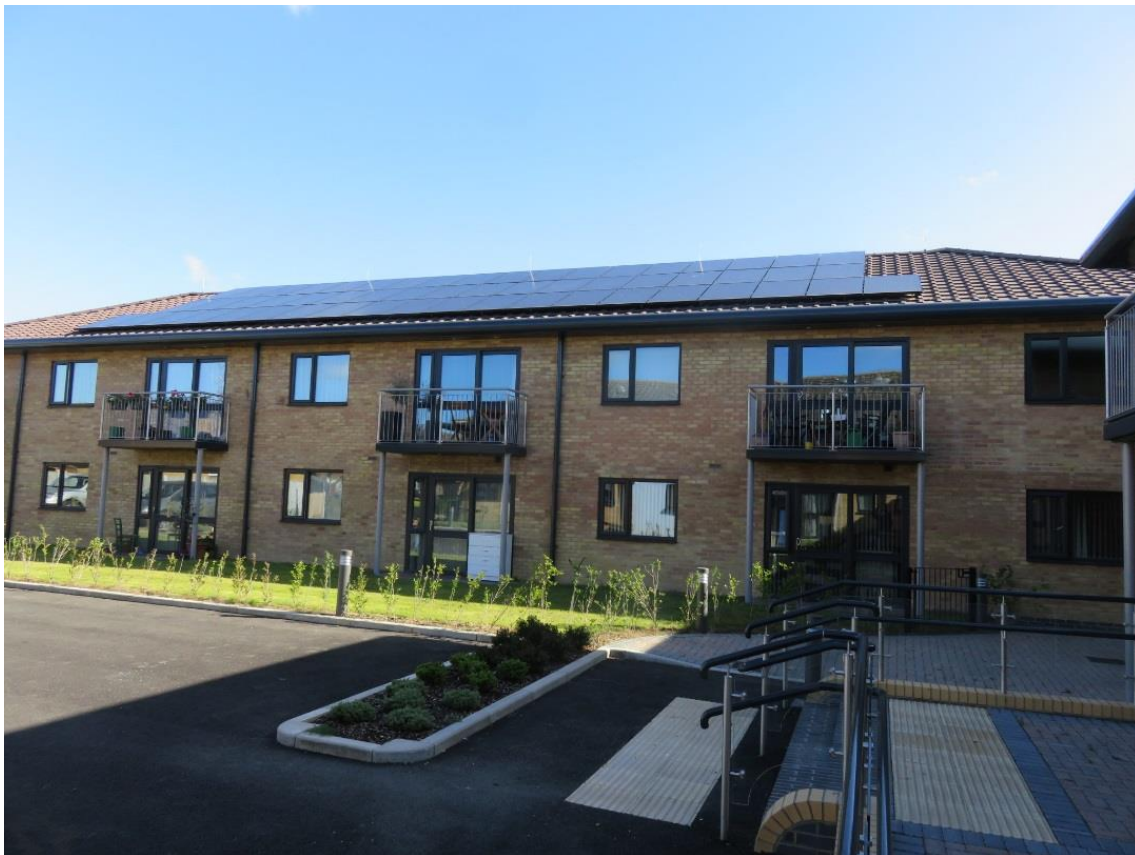
Figure 1.1 Picture of the exterior South elevation showing part of the PV array
