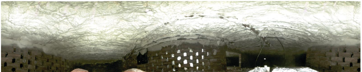
Figure 3.1 (d) Images of the resulting spray foam insulated floorboards from the under-side
