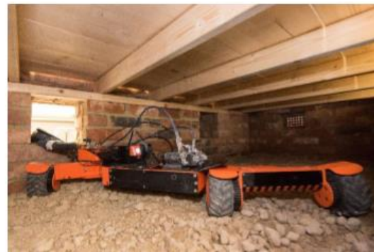
Figure 3.1 (b) Q-Bot being inserted into the under-floor space
