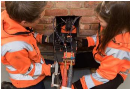
Figure 3.1 (b) Q-Bot being inserted into the under-floor space
