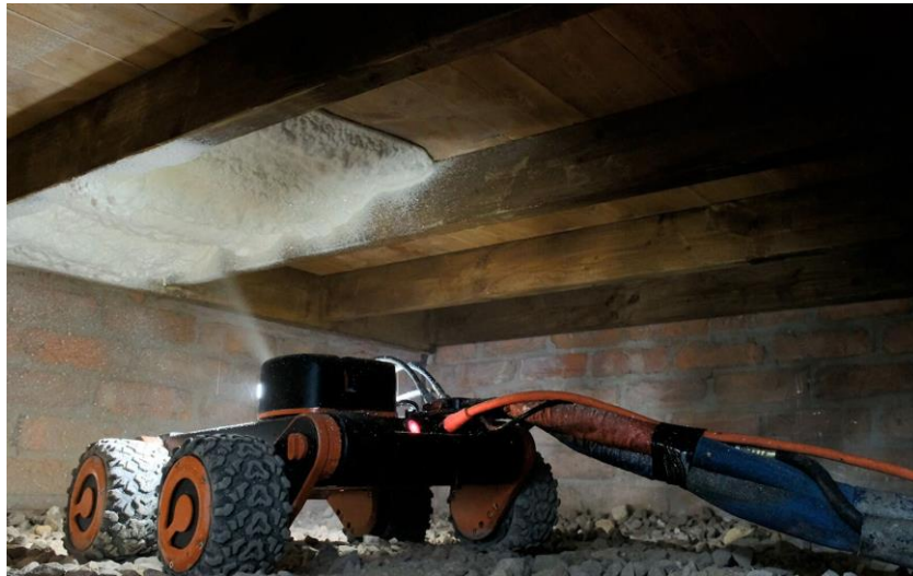
Figure 3.1 (d) Application of insulating spray foam to the under-side of floorboards using the SprayBot
