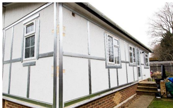
Figure 3.2 Schematic and photograph showing ‘tophat’ rails fitted on the walls and around the windows of a park home 19
