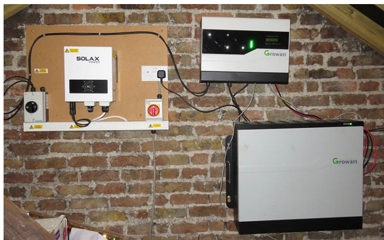
Figure 3.6 Installation with a Growatt SP2000 controller and GBLI5001 battery
