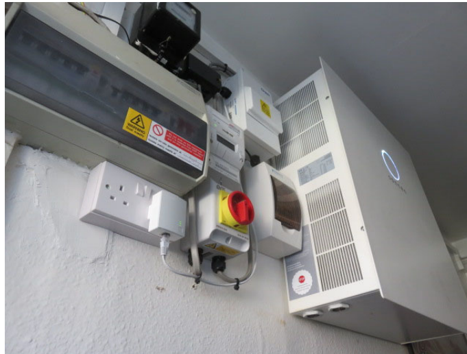
Figure 3.5 sonnen 2kWh battery installed in the hallway of one of the homes
