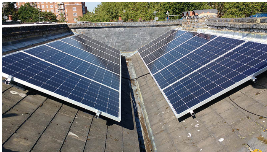
Figure 1.3 Solar PV installation on a property in Camden with a London Valley roof
